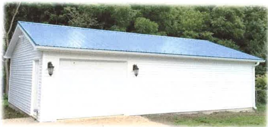
St. John's Lutheran Church Multi-Purpose Shed Constructed by Olson Home Improvements, LLC
